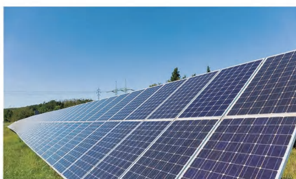
Yuzhou Peak Photovoltaic Power Station Project
