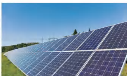
Yuzhou Peak Photovoltaic Power Station Project
